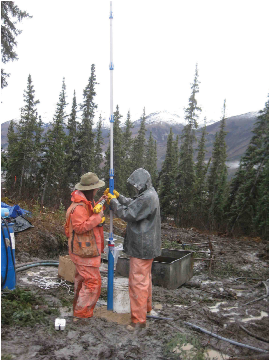
Figure 2. Installing the INC500 within the guide casing (photograph courtesy of J. Simpson).
